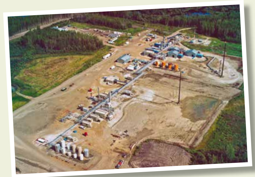
The Chinchaga operation in 2002. Chevron discovered this gas field in northwestern Alberta in 1981.
