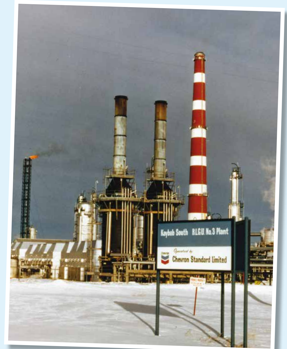
The Kaybob South Gas Plant, September 1977.
