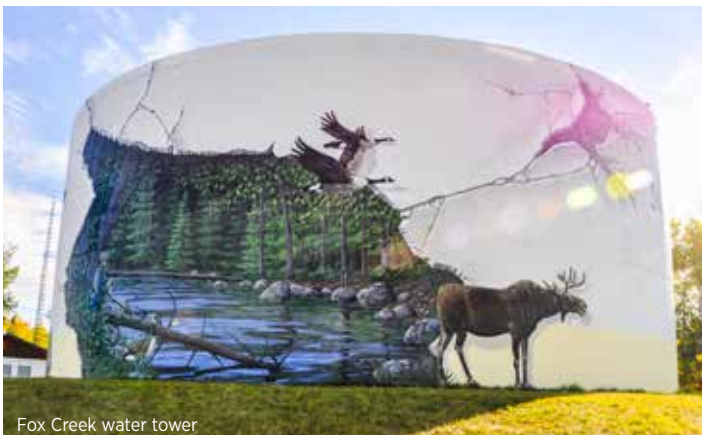
Fox Creek water tower
